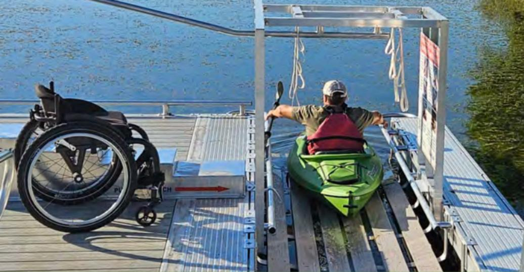
The adaptive kayak and canoe launch at Lake Chaminwood assists paddlers as they head out onto the water. It includes pull bars that allow users to pull themselves down the chute.
