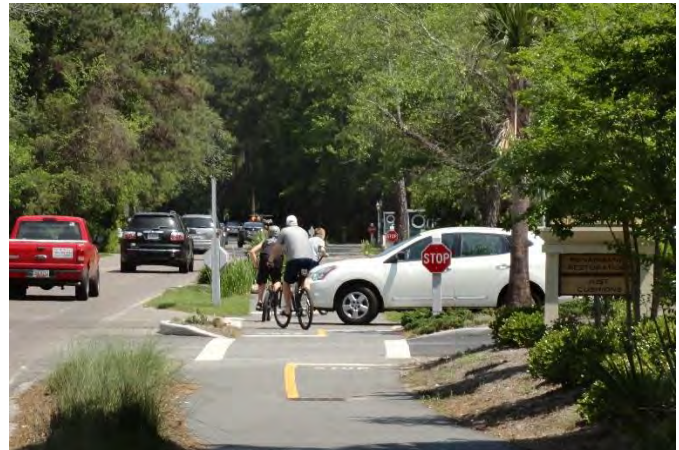
Sidepaths can present conflicts between people bicycling and people driving, especially at intersections and driveway crossings (above). Steps can be taken to mitigate these conflicts. Examples include high-visibility pavement markings, specialized warning signs, and enhanced traffic signals (below).
